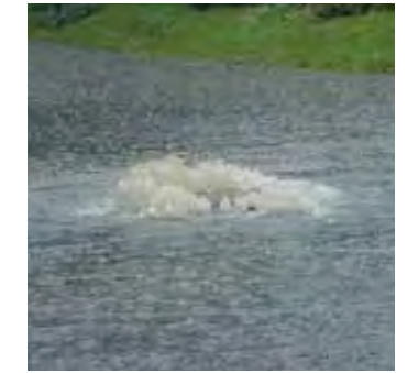
Sewer manhole overflowing in New Paltz, NY due to aging infrastructure that combines both stormwater and sanitary sewer. Photo credit: Scott Cuppett
